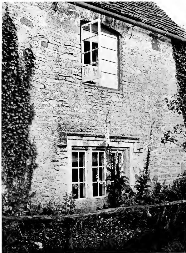
DETAIL OF COTTAGE AT COTSWOLD HILLS
